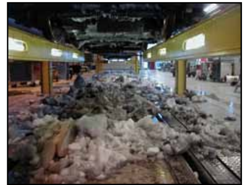
Costly. Before the installation of the Nordic systems. Several tons of ice to de-ice. It will take several hours before the train is back in service.
