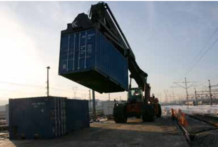
Successful winter installation in Alnabru, Norway.
